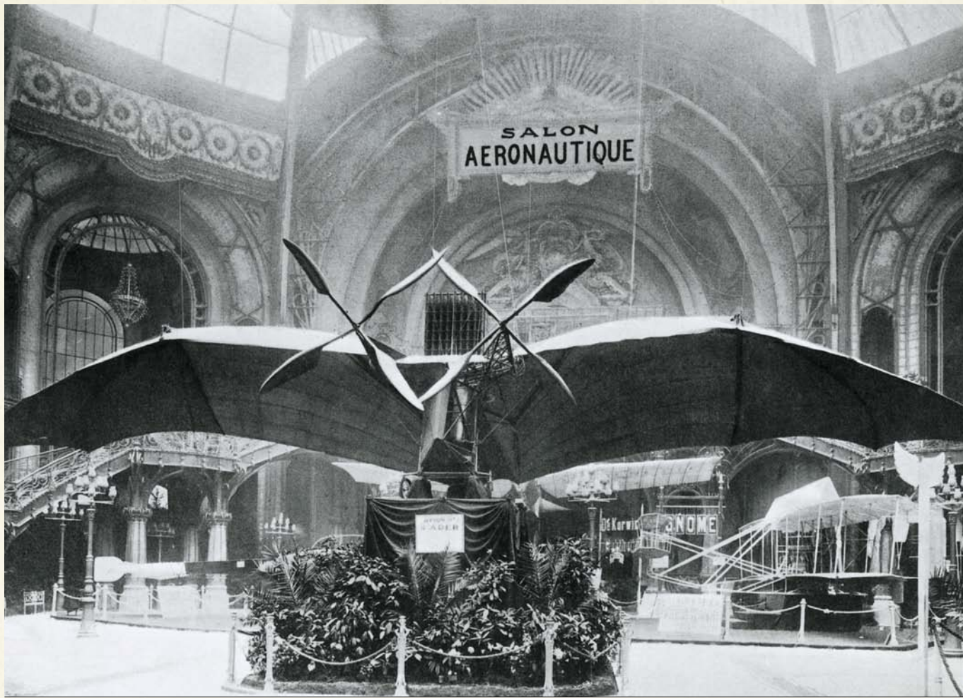
ADDER MODELLED HIS CURIOUS STEAM-POWERED MONOPLANE ON THE BAT
