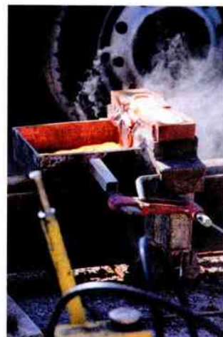
Welding railway rails using an exothermic reaction.
