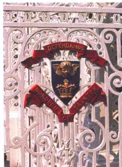
The paint on this park gate stops it from rusting.
