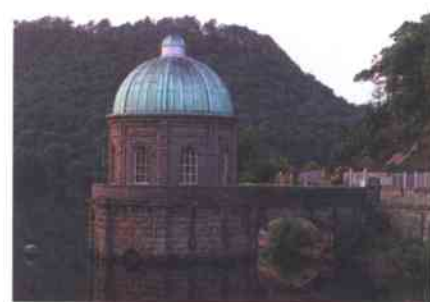
Changes in all metals, such as when a copper roof turns green, are chemical changes but they are not called rusting.
