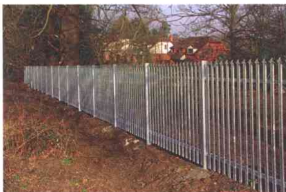
The layer of zinc on this fence stops it from rusting.
