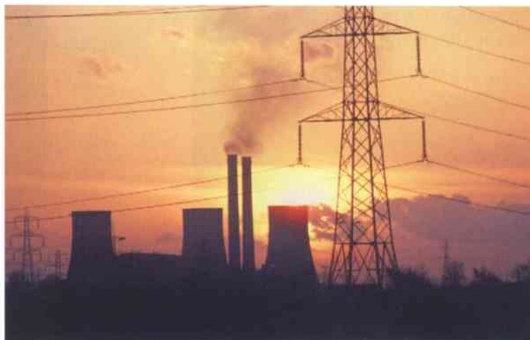
The electricity produced by this power station is carried away in cables hanging from the tall pylons.
