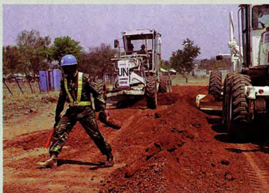
An infrastructure project – ditch-digging
