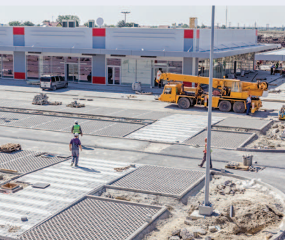
Building a new supermarket
