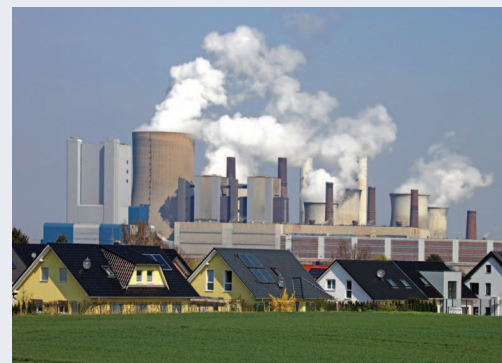
A power station
