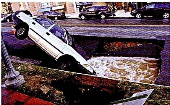
A car falls into a sinkhole
